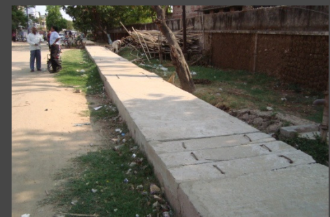
Completed lateral Drains
